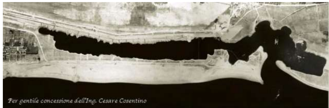
Gioia Tauro harbor under construction. Note the dredges at work within the basin and the barge disposing at sea the dredged material, just outside the harbor entrance, where a landslide will occur on 12/7/1977
